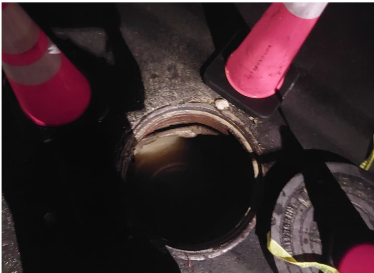
Image: 20230721_225142 – Debris Removal Work Zone
