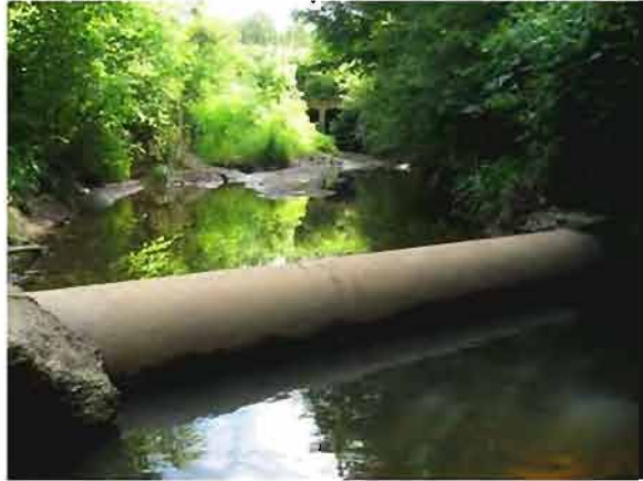
Site 25. Pipe Crossing at the waterline.
