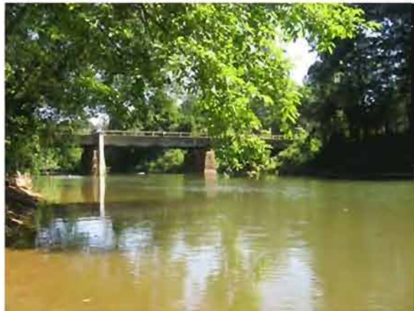
Site 136. View of Klondike Road Bridge.
