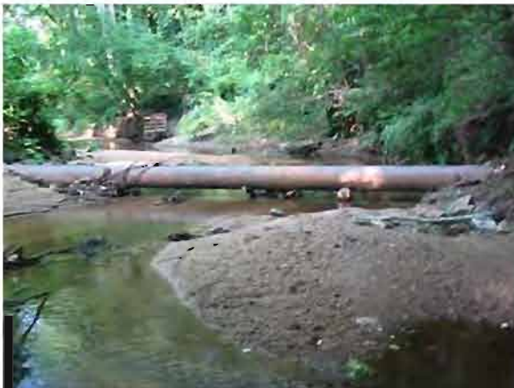
Site 71. Pipe crossing at the waterline.
