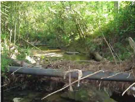
Site 14. Pipe crossing above the waterline.
