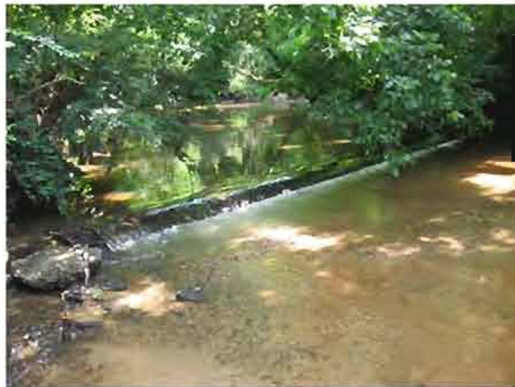
Site 55. Pipe crossing below the waterline.
