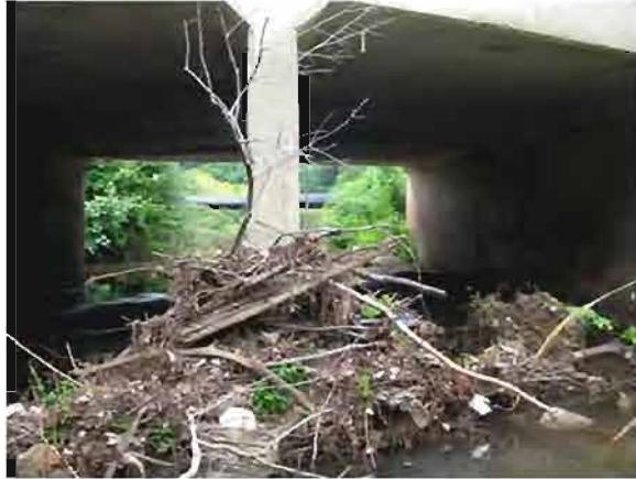
Site 68. Box culvert under Park Drive.
