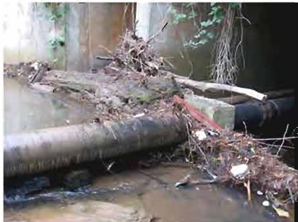
Site 66. Pipe crossing at the waterline.
