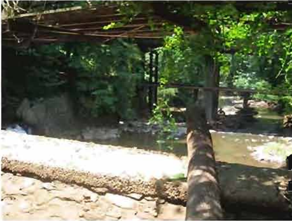
Site 58. View of concrete and stone dam.
