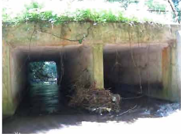
Site 8. Box culverts under Elmdale Road.
