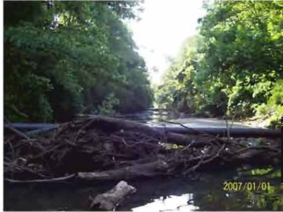
Site 120. Pipe crossing above the waterline.
