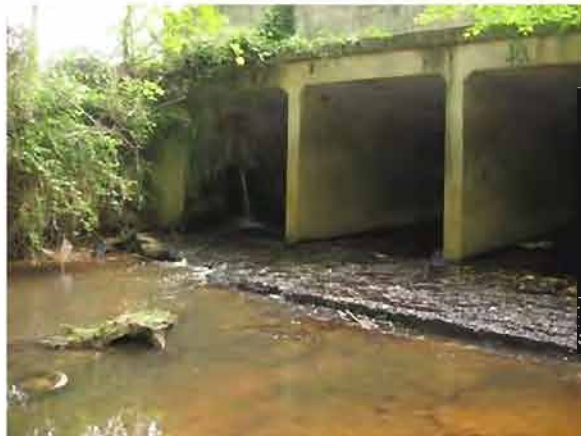
Site 40. Box culvert under Valley Brook Road.
