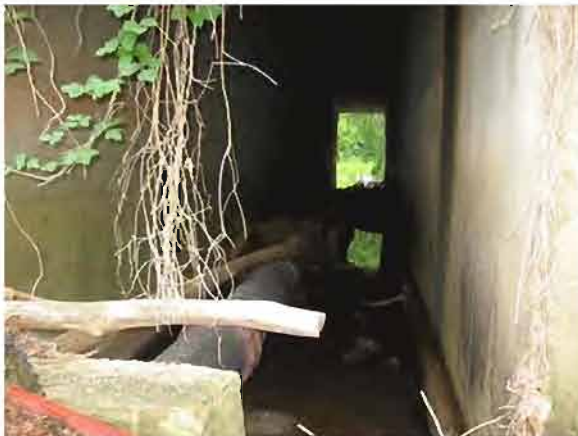
Site 66. Box culvert under Memorial Drive.
