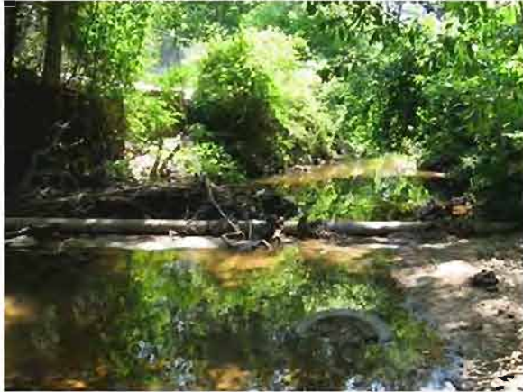
Site 30. Pipe crossing at the waterline.
