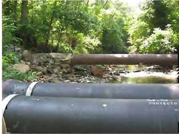
Site 53. Multiple pipe crossings of the stream.
