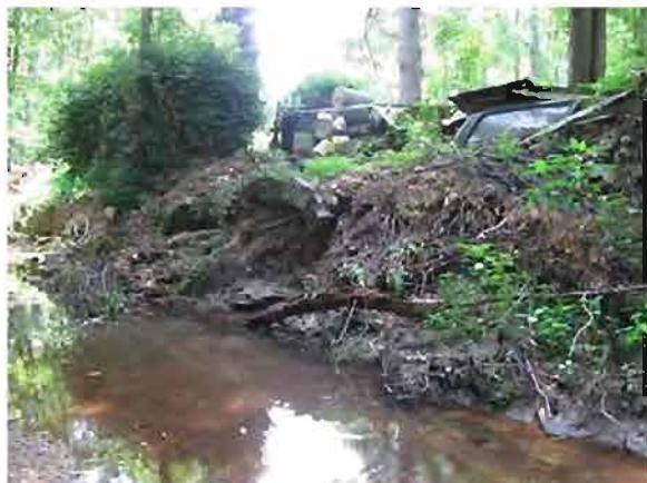
Site 17. Drum storage along the stream bank.
