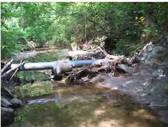
Site 16. Pipe crossing above the waterline.
