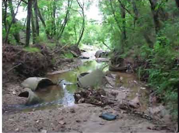
Site 13. Sections of RCP in stream.
