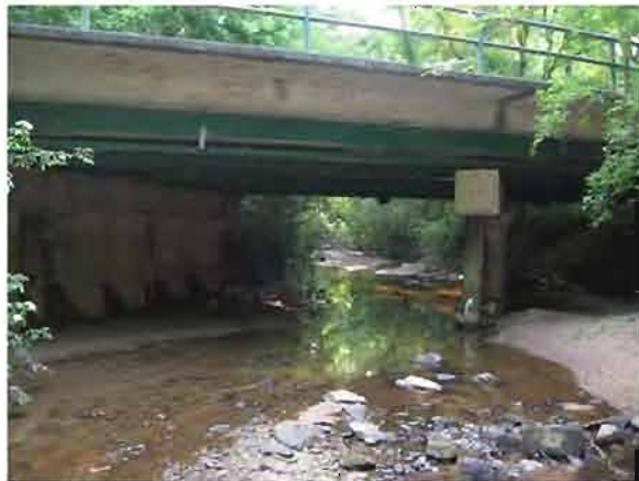
Site 33. View under Creekdale Drive Bridge.
