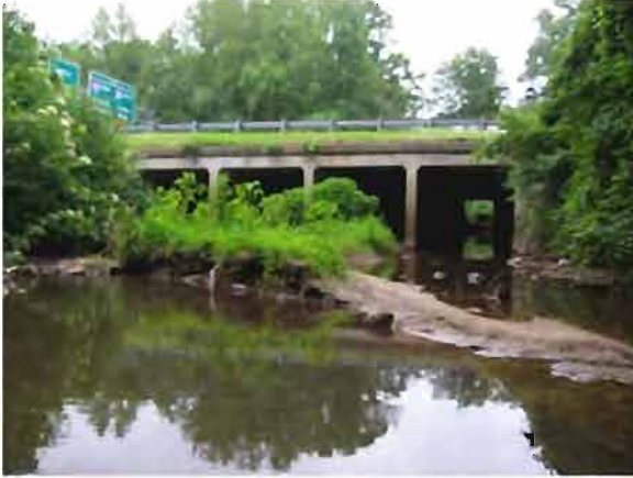
Site 36. Box culvert under Interstate 285.
