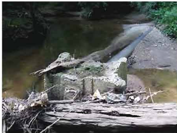
Site 27. Pipe crossing at the waterline.
