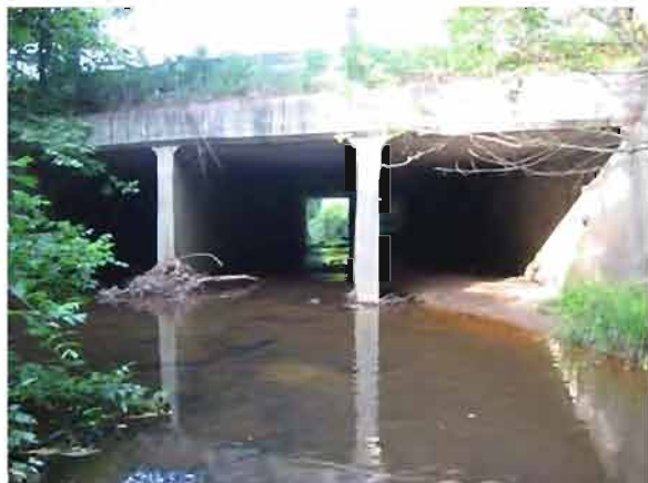
Site 23. Box culvert under Post Oak Drive.
