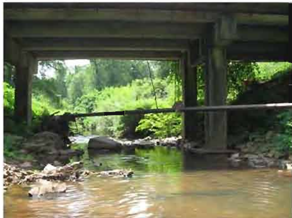
Site 82. View under Rowland Road Bridge.
