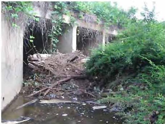
Site 32. Box culvert under Casa Drive.
