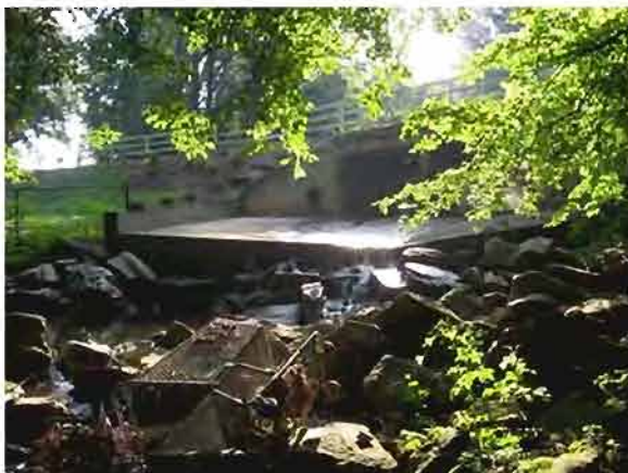
Site 22. Box culvert under Post Oak Drive.
