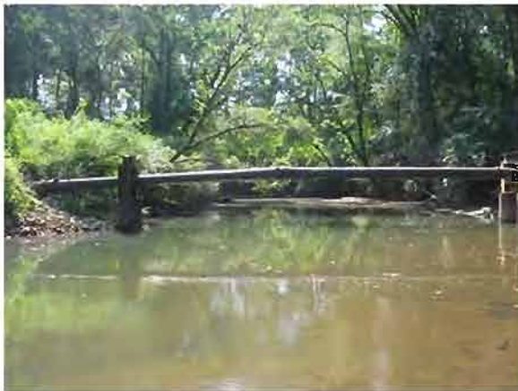
Site 127. Pipe crossing above the waterline.
