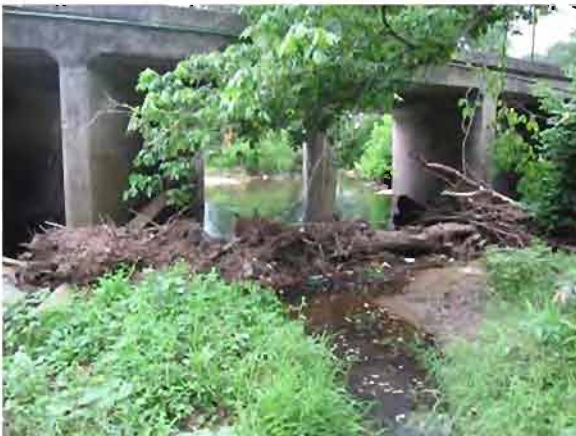
Site 39. Box culvert under Cedar Creek Drive.
