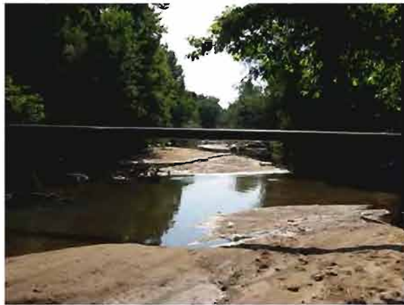
Site 116. Pipe crossing above the waterline.
